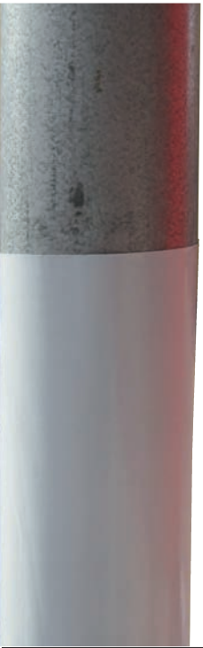
Film protects downpipes (e.g. during plastering)
